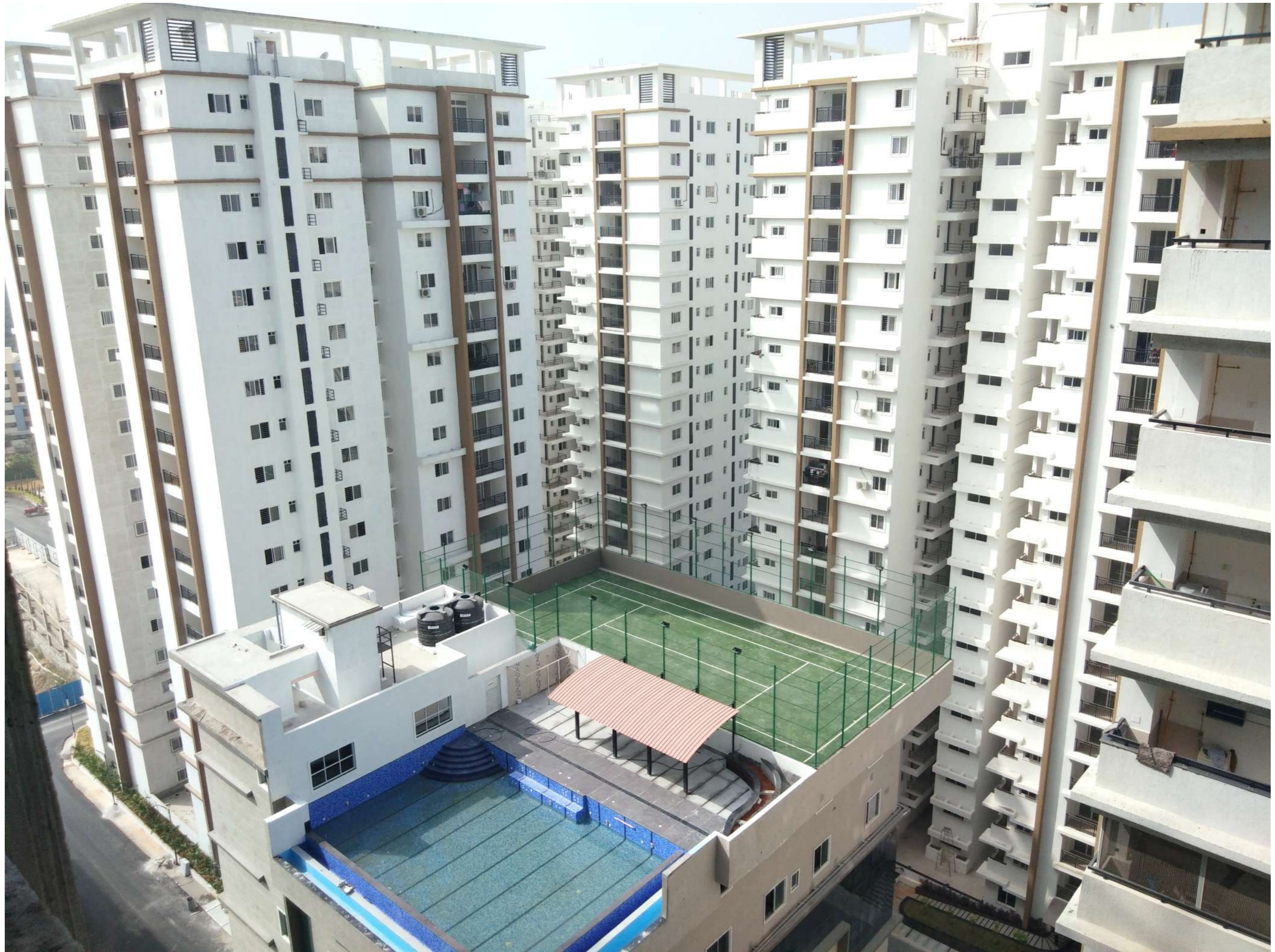
Roof Top Swimming pool with Tennis Court in ICONIA Clubhouse
