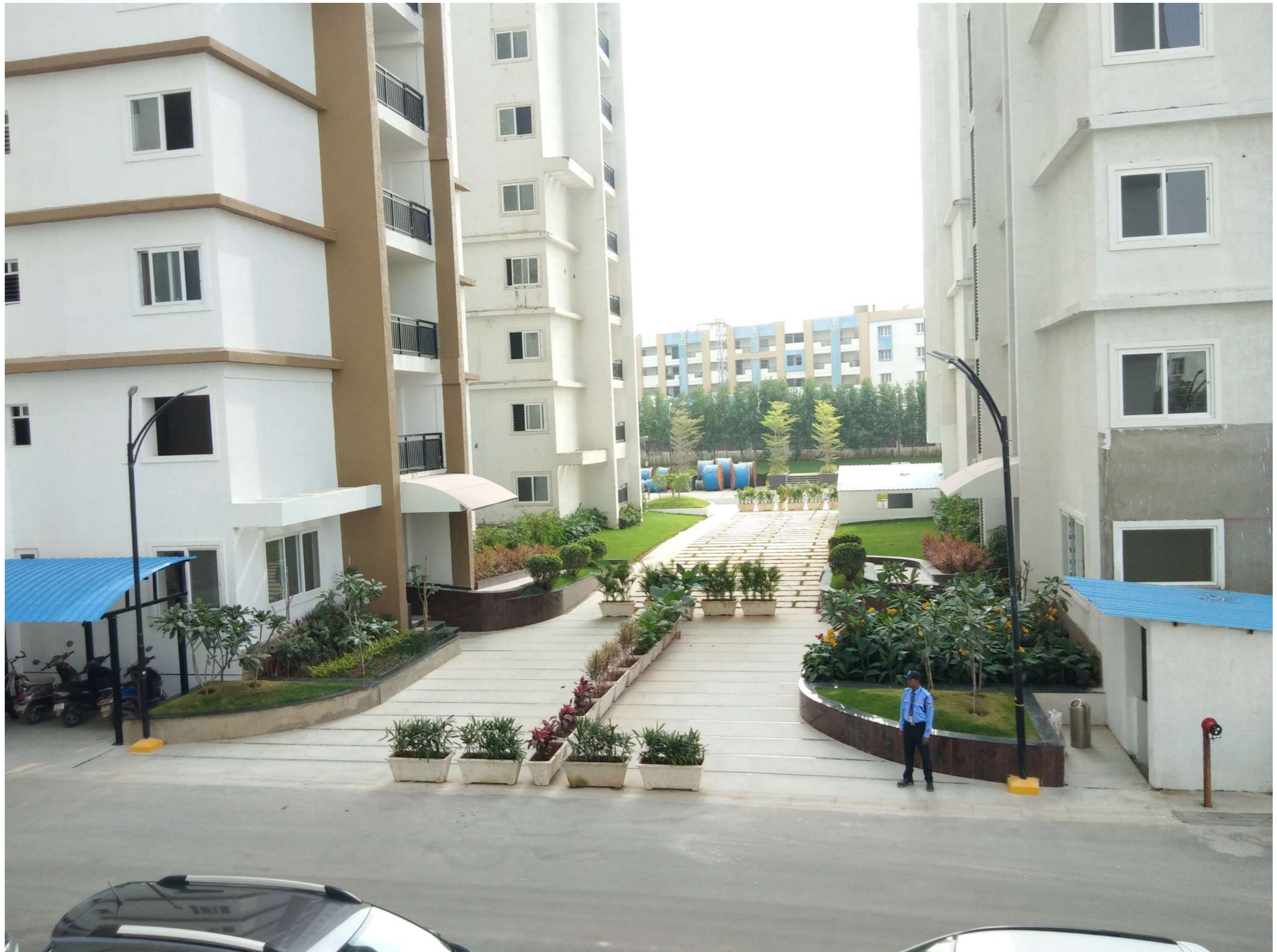
A Walkway Between the Block A & B in Phase - I
