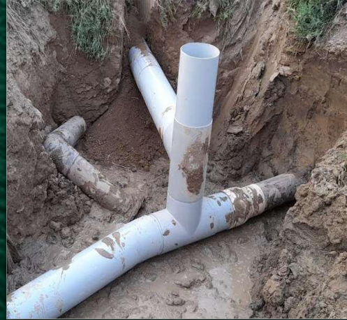
UNDERGROUND WATER PIPE LINE
