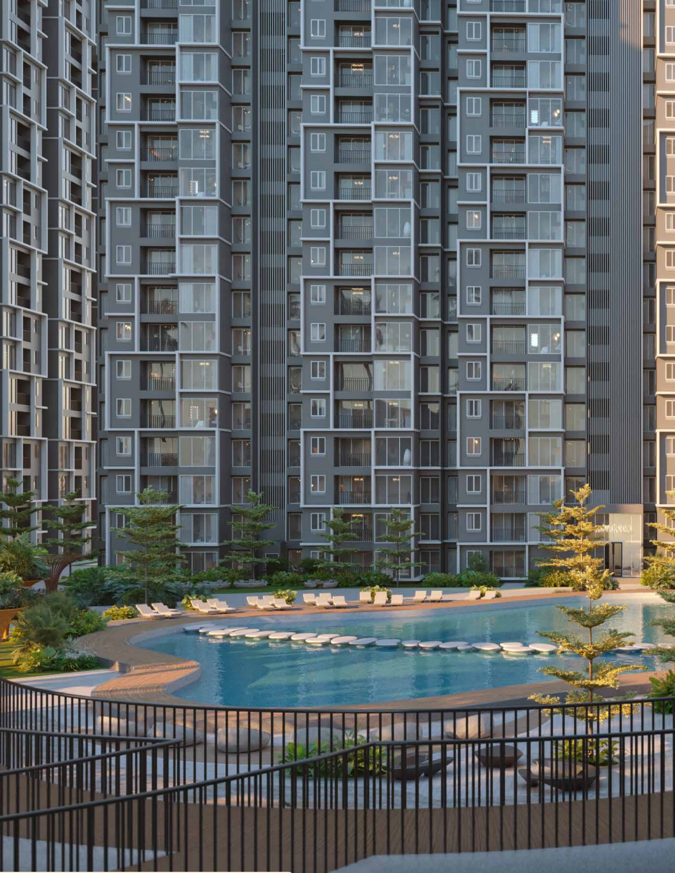
ELEVATION AERIAL VIEW
