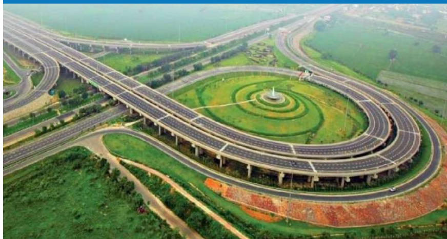
MUMBAI - DELHI EXPRESSWAY
