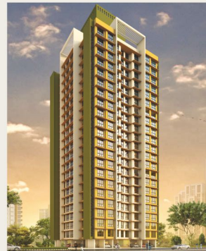
ADITYARAJ AVENUE VIKHROLI
