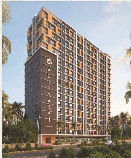
ADITYARAJ SPRINGS CHEMBUR
