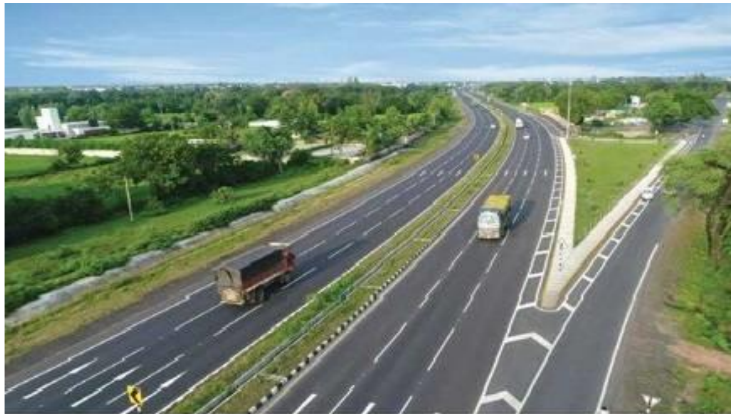
PANVEL-BHIMASHANKAR ROAD CONNECTOR - 50% WORK COMPLETED
