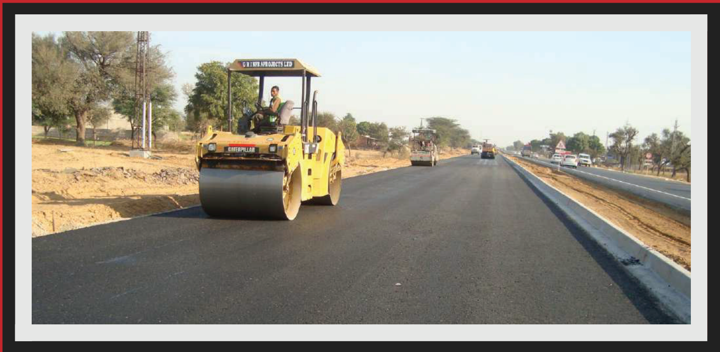
INTERCITY ROADS PROJECT MUMBRA, MUMBAI
