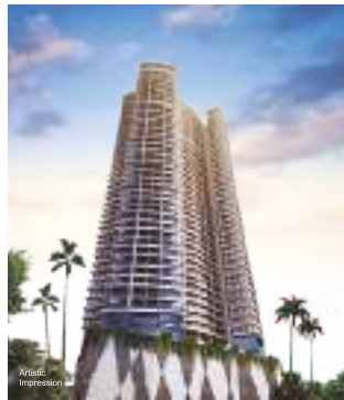
J P DECKS, GOREGAON (EAST)
