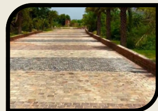
Roads With Interlocking Tiles
