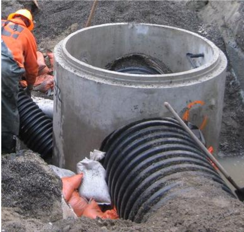
UNDERGROUND SEWERAGE LINE
