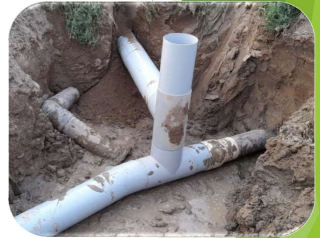
UNDERGROUND WATER PIPE LINE
