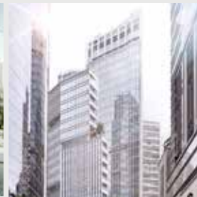
Bamboo Towers, Malaysia
