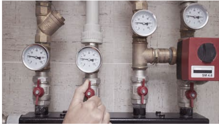
Smart Metering for Water and Electricity
