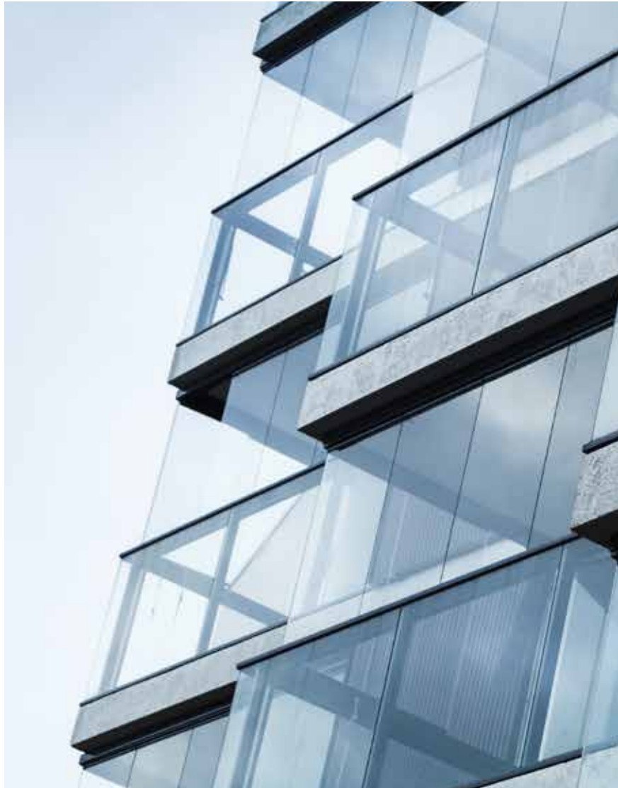
High-performance Glass Facades to Reduce Heat Gain
