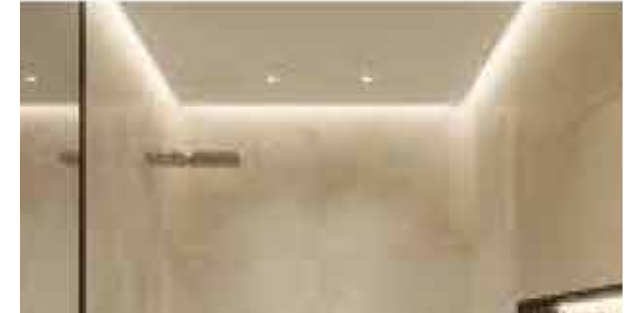
Acrylic Emulsion Paint on Ceiling & False Ceiling
