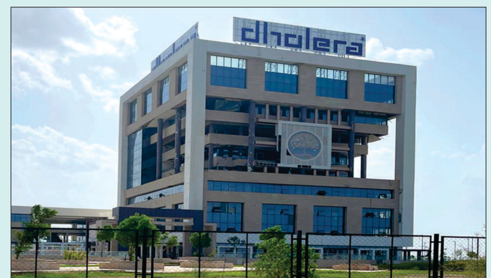
ABCD BUILDING - DHOLERA SIR
