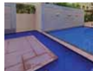
20 Floating Deck in Reflection Pool
