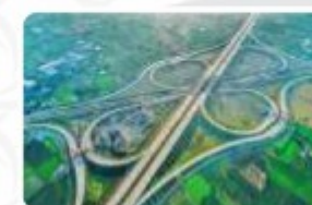
Eastern Peripheral Expressway
