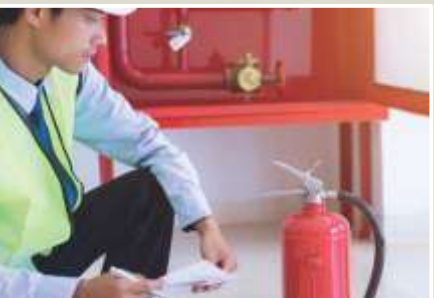
Fire Fighting System in Each Flat
