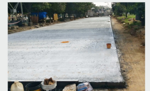
Cement Concrete Road
