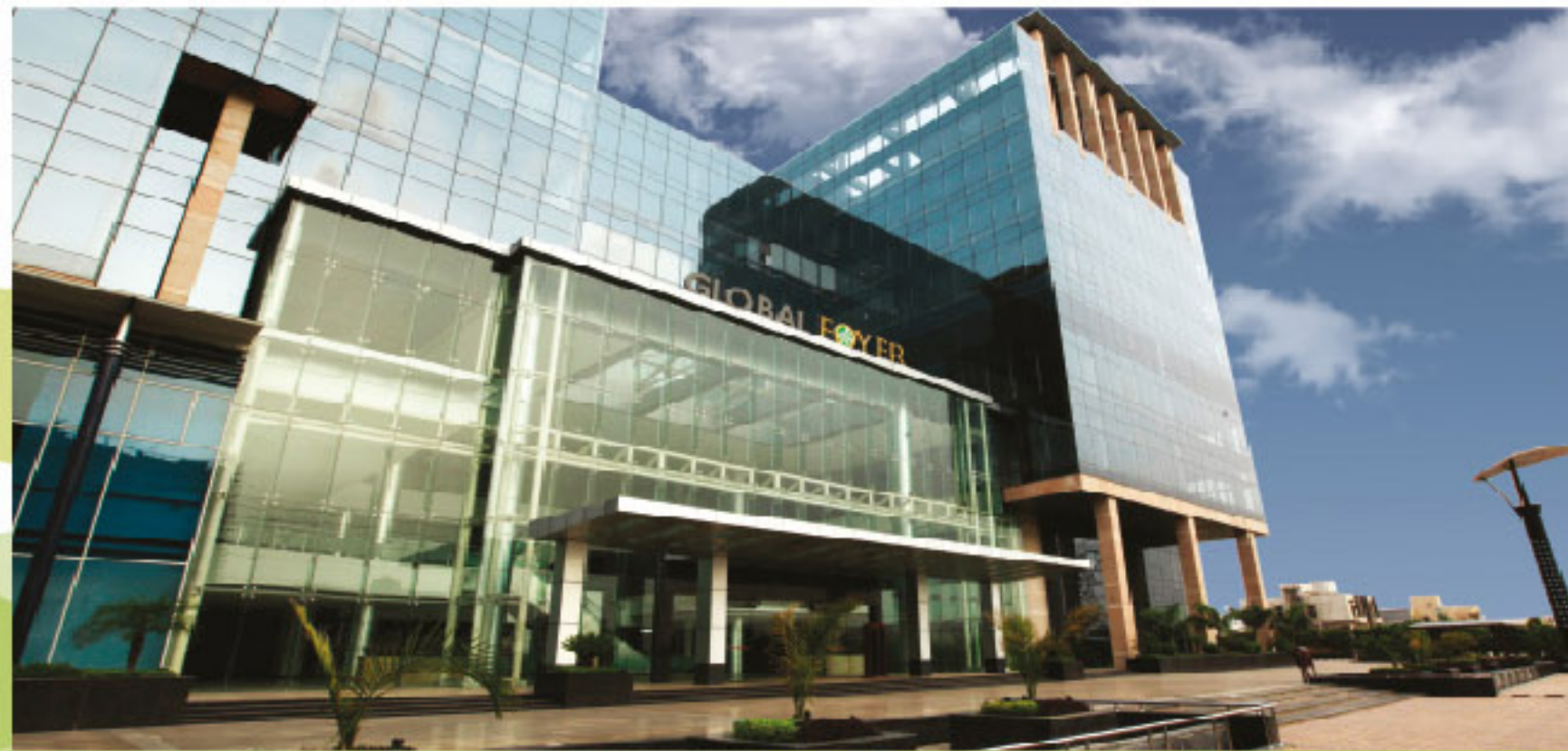
Global Foyer, Gurgaon
