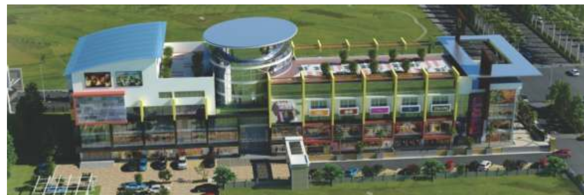
Covent Court - Satna (Ongoing Project)
