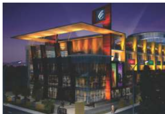
Covent Court - Satna (Ongoing Project)
