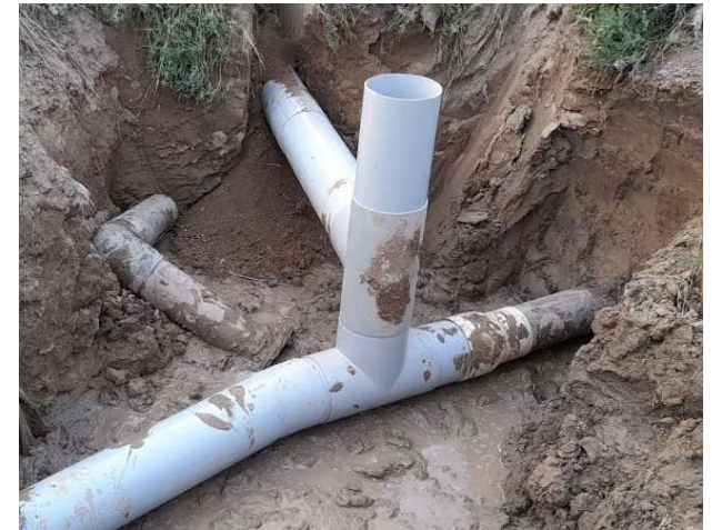
UNDERGROUND WATER PIPE LINE
