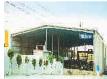
BCC PRECAST PLANT
