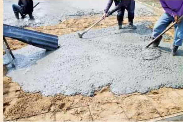
Premix mixes into the fluid concrete mixture which is then sprayed.
