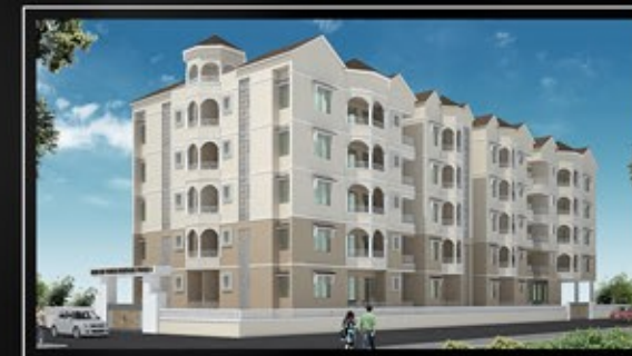
Hari Om Tower Heritage Phase II Ranchi
