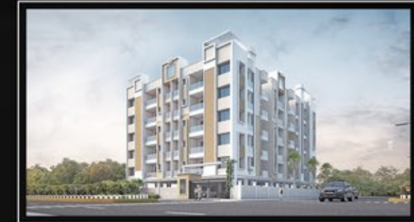
Mira Tower I Ranchi
