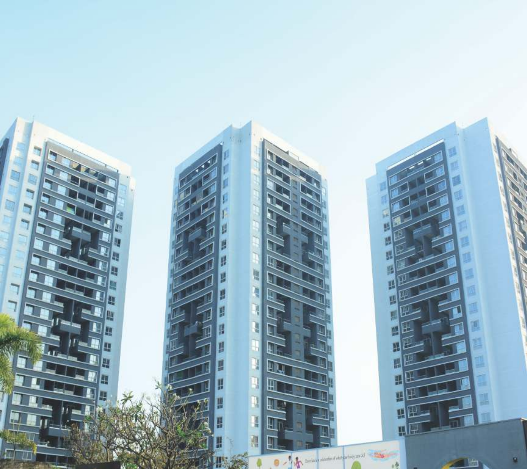
Completed Phase 1- A, B & C Towers
