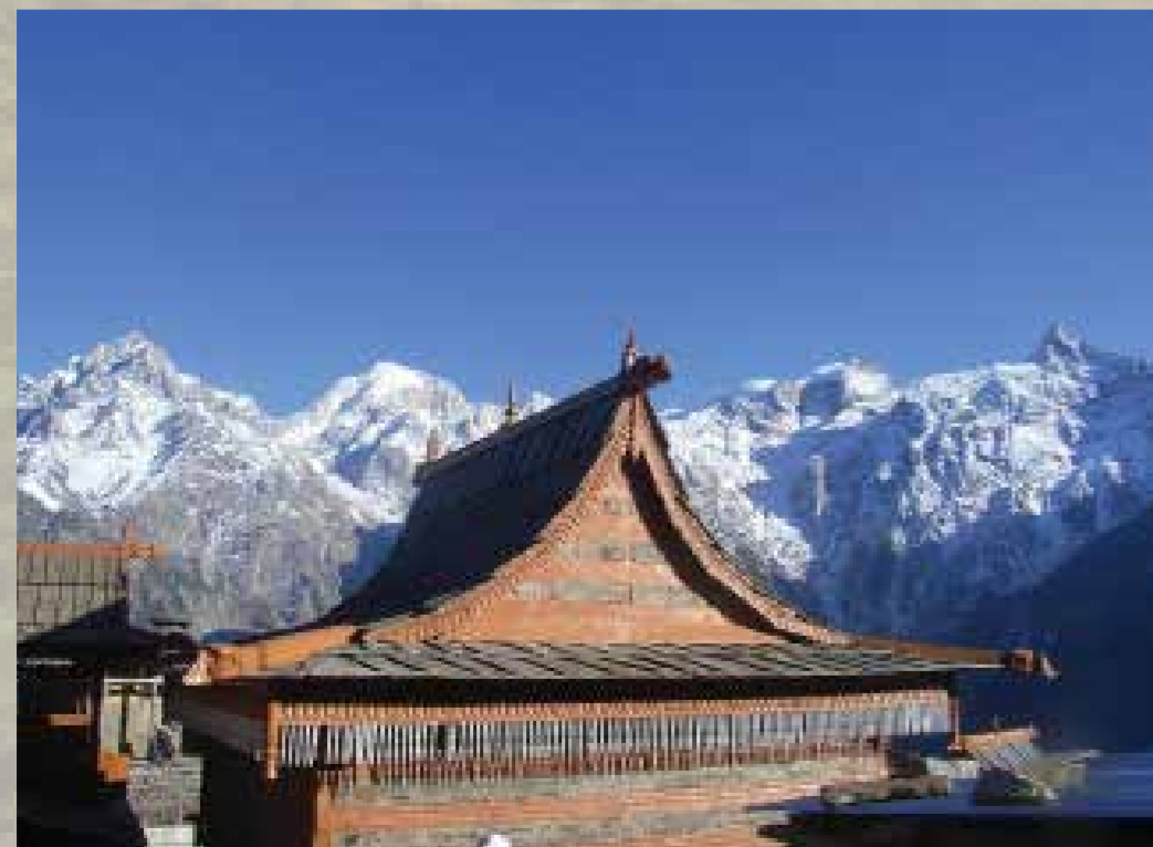
Signature Himachali roof detailing that is reminiscent of the Himalayan peaks.
