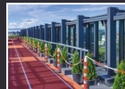
YOUG TRACK ROOF TOP
