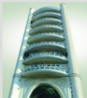
Buckley Court COLABA
