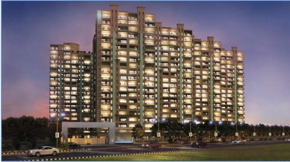
Pareena Coban, Sector 99A, Gurugram 1.3 Million sqft; Phase 1 to be delivered in 2022
