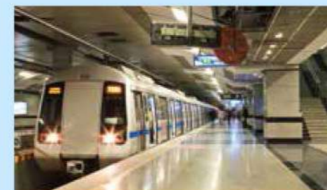
Barakhamba Underground Metro Station - New Delhi
