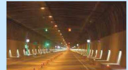
Chenani-Nashri Tunnel - Jammu & Kashmir
