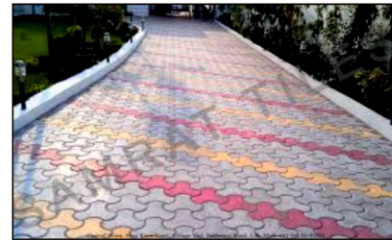
INTERLOCKING TILES ROAD
