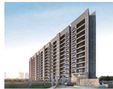
THE NEW DOOR SEZ, Ajmer Road
