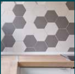
DADO CERAMIC TILES 600 MM ABOVE THE COUNTER
