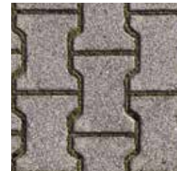
INTERNAL ROADS INTERLOCKING BLOCKS/ TREMIX CONCRETE ROAD
