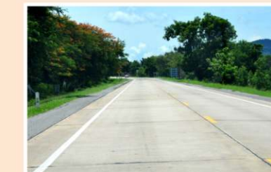
Internal Concrete Road
