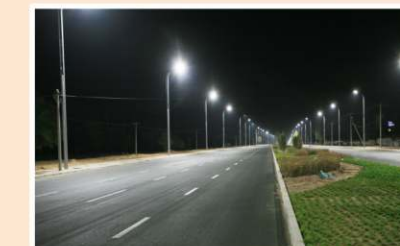
Electrification With Street Lights
