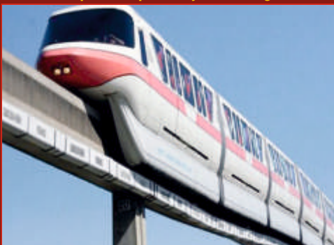
Rapid Rail Delhi to Meerut in Front of Project, NH-58 (Work Started)
