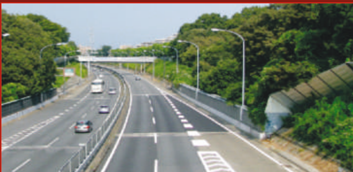
Eastern Peripheral Expressway Connecting Palwal-Ghaziabad-Delhi Just 700 Mtr.
