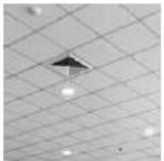
CEILING GRID FALSE CEILING
