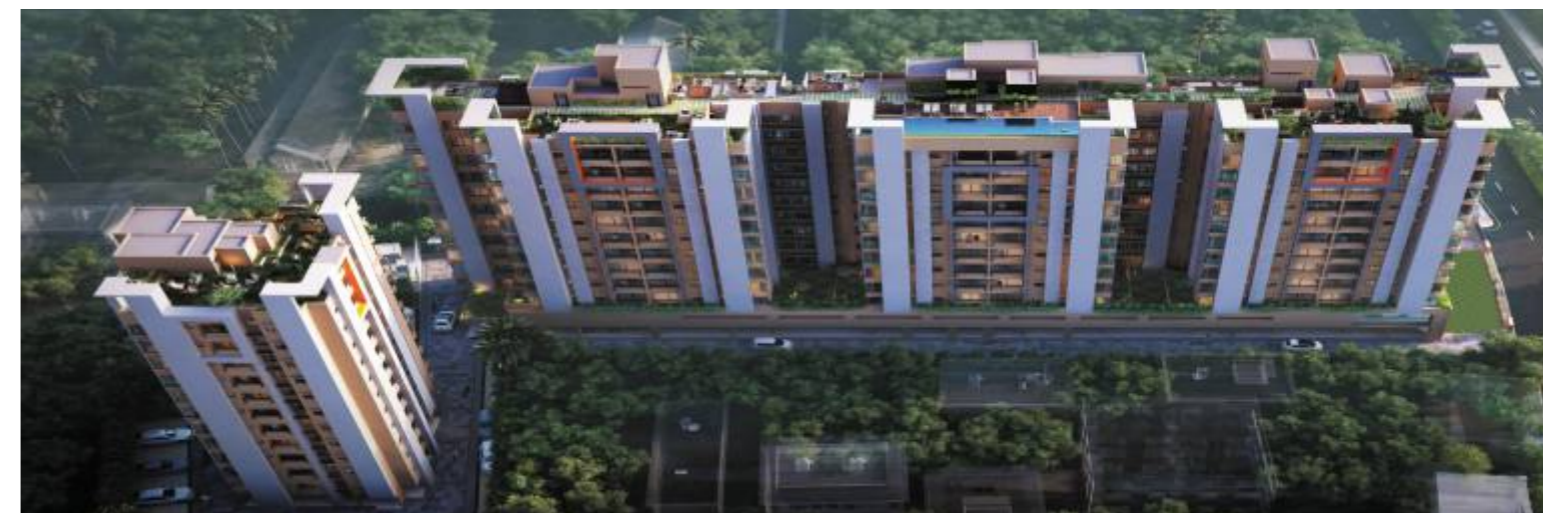
RISHI VENTOSO, Madhyamgram, Kolkata (Under Construction)
