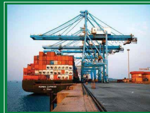
JNPT: ▲ INDIA'S LARGEST CONTAINER PORT
