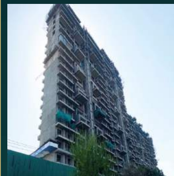
STRUCTURE & BLOCKWORK COMPLETE: TOWER A & B
