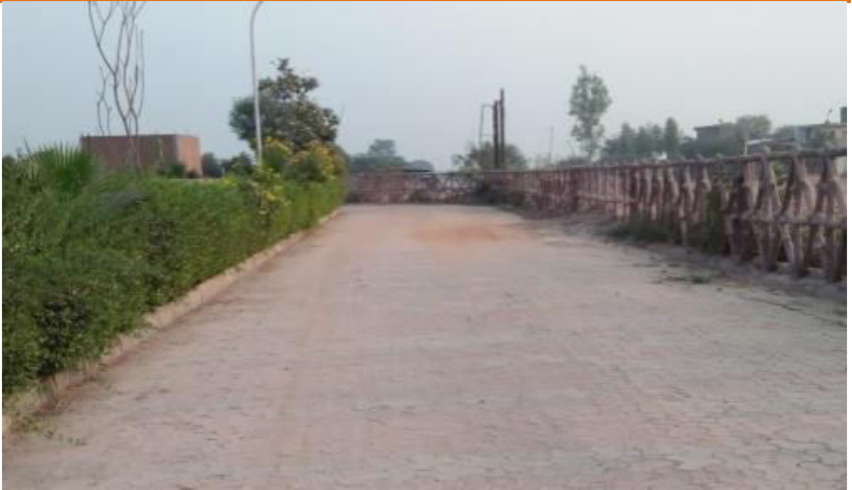
Wide Concrete Road
