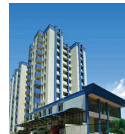
Shirdi Phase 1 Opp St. Thomas School, Trivandrum
