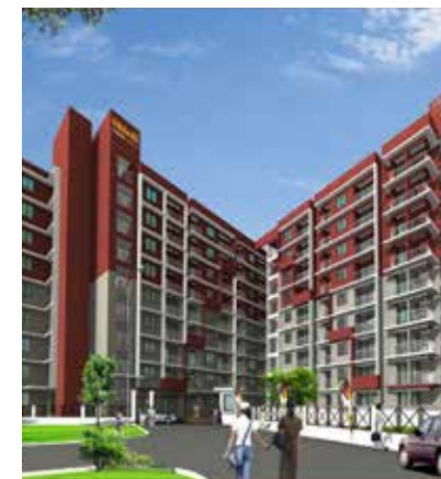
Shirdi Phase 2 Opp St. Thomas School, Trivandrum
