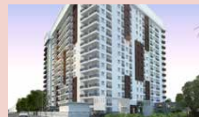
Sowparnika Columns, Bangalore
