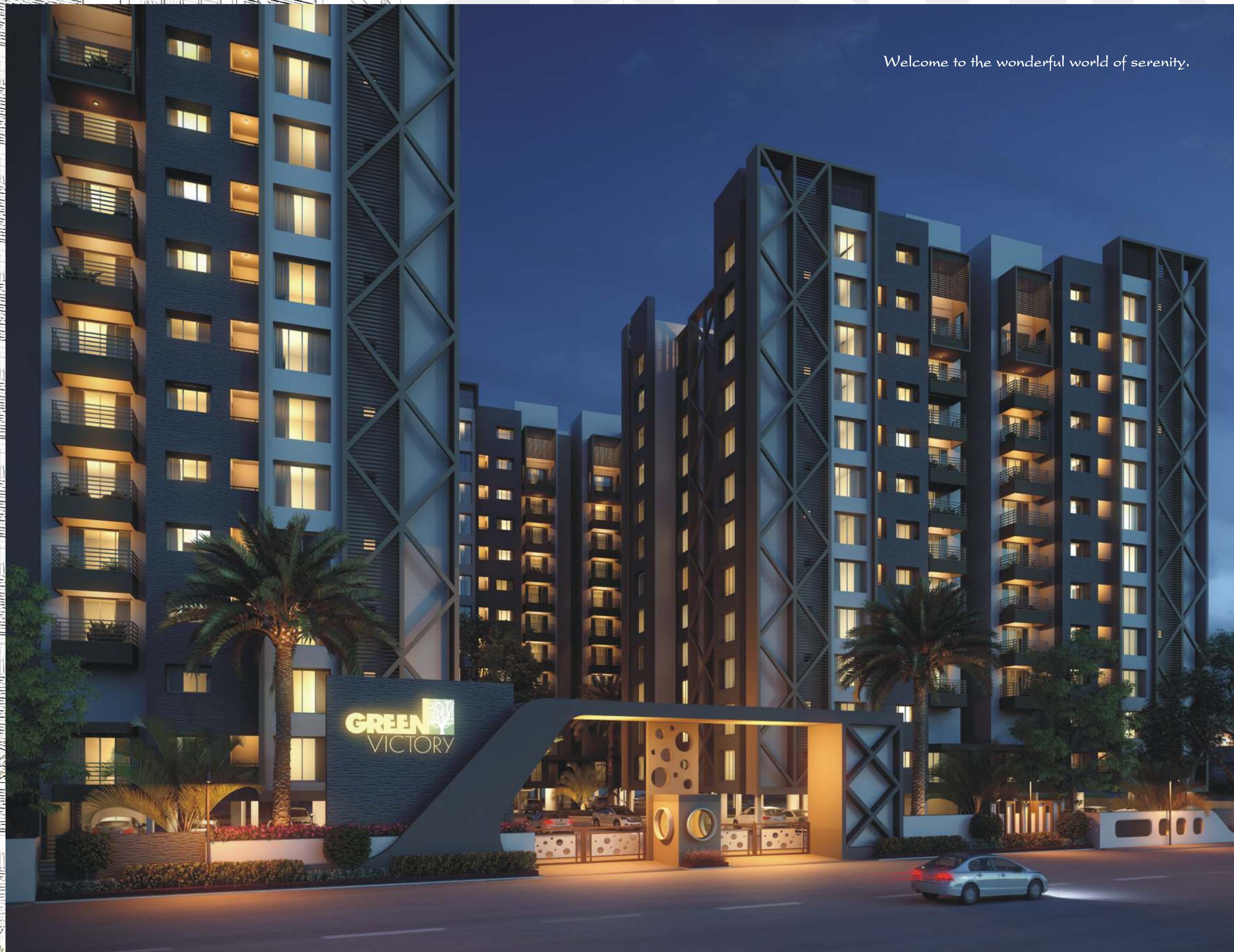
Main Entrance gate
