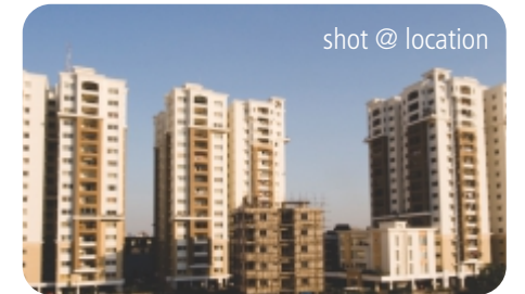
Fortune Towers @ Hyderabad
