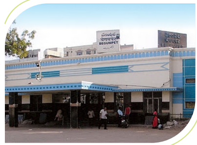
Begumpet Railway Station
