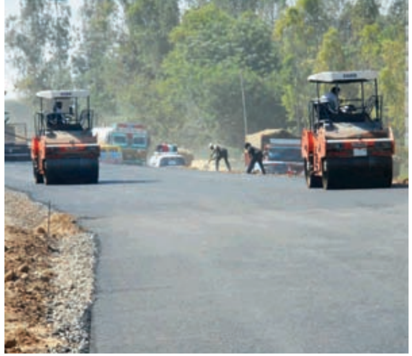
EXISTING 4 LANE HIGHWAY DEVELOPMENT WORK IN FULL SWING
