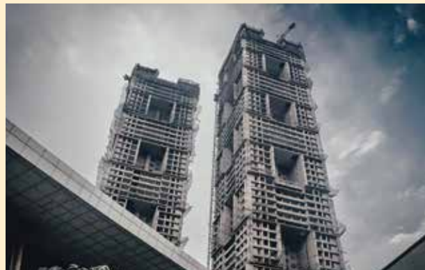
Actual View of the Iconic Towers
