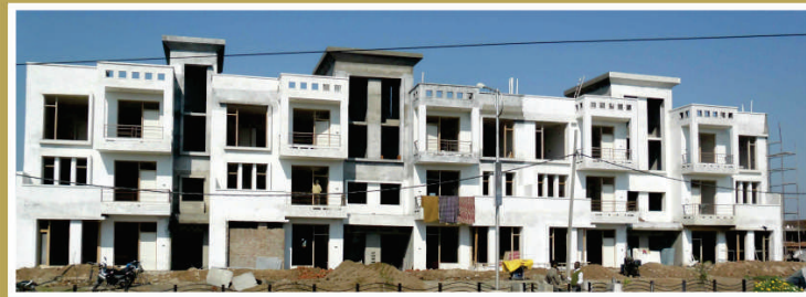
'TDI Complete Homes' nearing Completion
