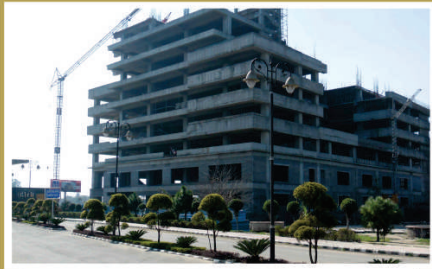
'TDI Business Centre' under Construction
