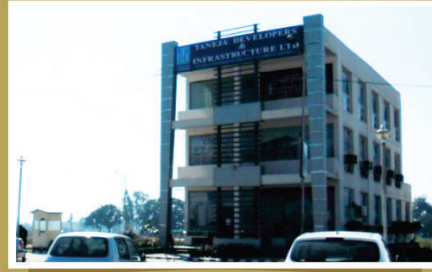
Commercial Plots already delivered & are under construction
