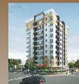
GOVIND REGENCY Tilak Nagar, Jaipur
