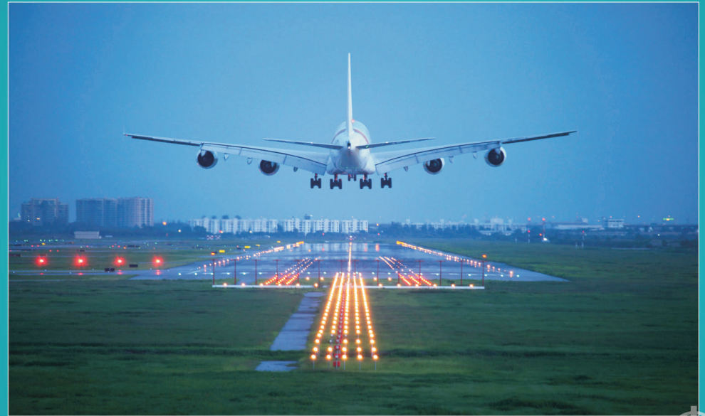
Indira Gandhi International Airport
