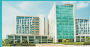
Medanta Hospital, Gurgaon
